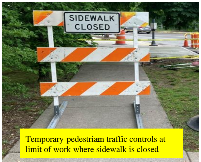
Temporary accessible sidewalk during construction
