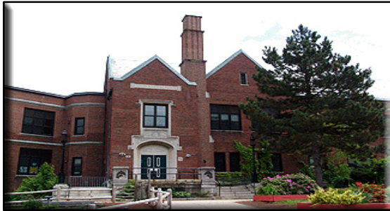
WARD ELEMENTARY SCHOOL
