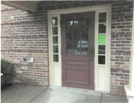
Photo 3 – View of a typical common entry door.
