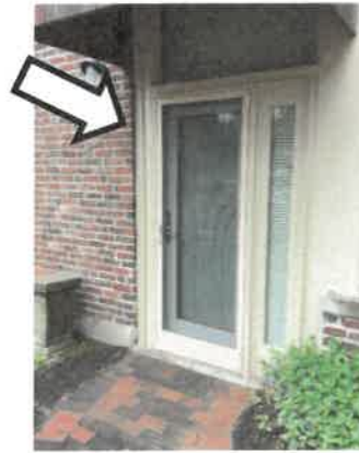
Photo 2 – View of a typical unit entry door.
