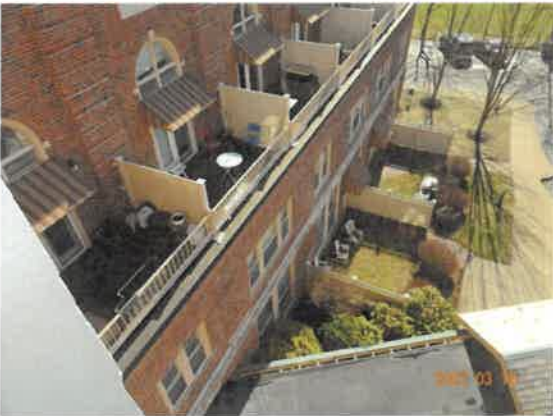
5. Typical view of the privacy fences. Good condition.
