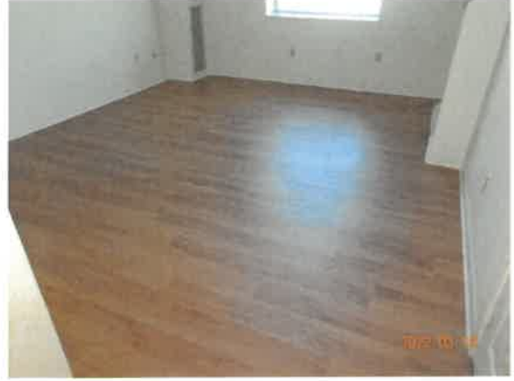
20. View of living area floor coverings.
