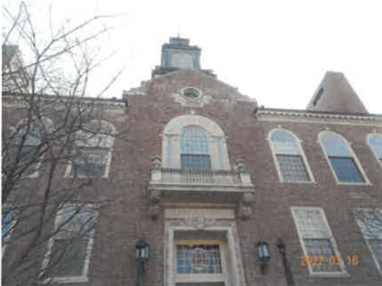
9. View of the front of the building. Decorative cast masonry in good condition.
