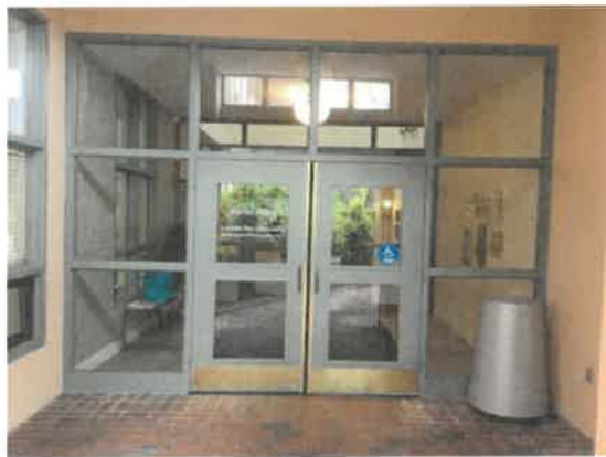
Photo 1 – View of the main entrance doors.
