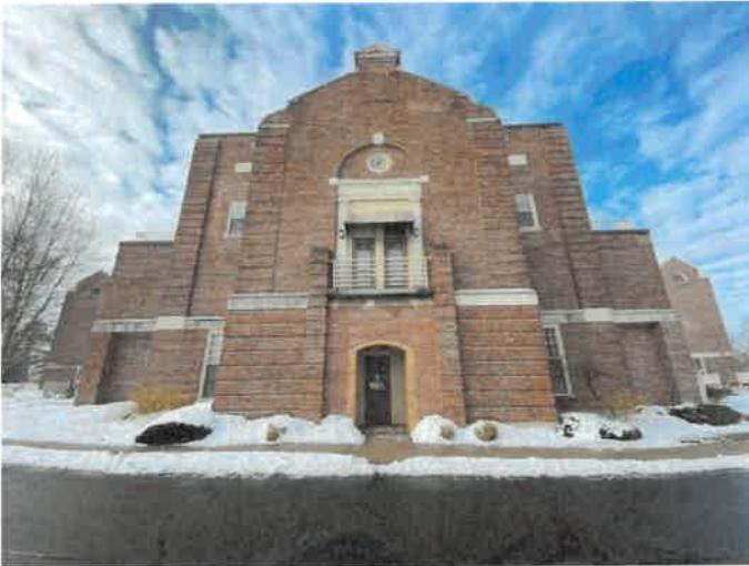
Photo 1: Overall partial view of the rear elevation of the Warren House where emergency sounding, and temporary repairs of the cast stone copings and other ornamental stone were performed.
