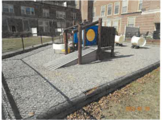
6. View of the playground at the back of the building. The playground is not on an accessible route.
