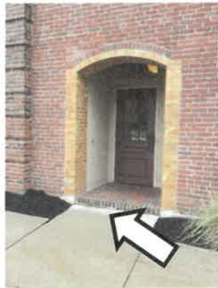
Photo 9 – View of the yellow glazed brick masonry.
