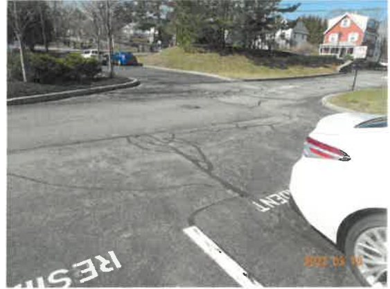
2. View of the entrance paved area. Note that the over-flow parking lot appears to be newer.
