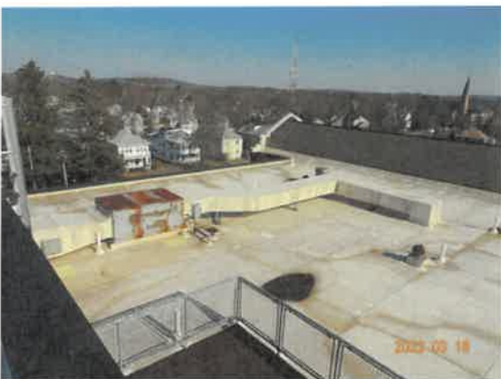
11. View across the TPO roof covering.
