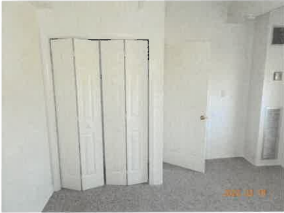
19. Typical view of the dwelling unit interior passage and closet doors.
