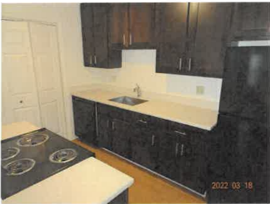
21. Typical view of the newer kitchen cabinets.
