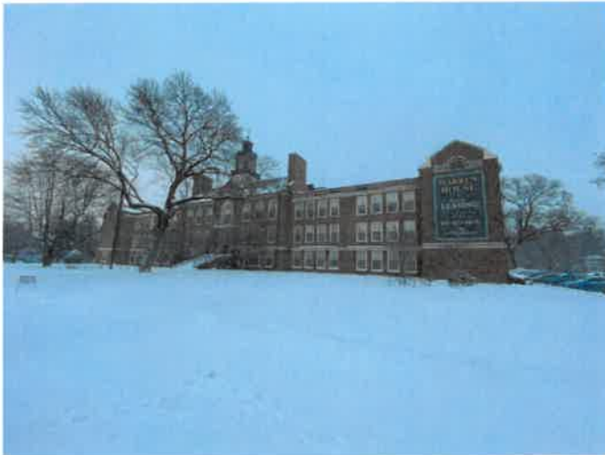
Photo 1: Overall view of the front elevation of the Warren House where emergency sounding of the cast stone copings was performed.
