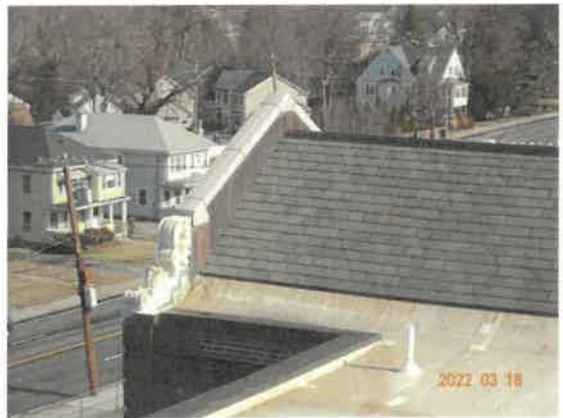
12. View of the slate roof covering. Good condition.
