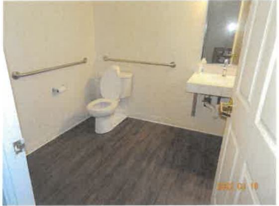
18. View of the common-use restroom.
