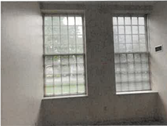
Photo 1 – Overall interior view of typical window units.
