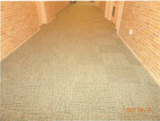
15. Carpet tile is in good condition.
