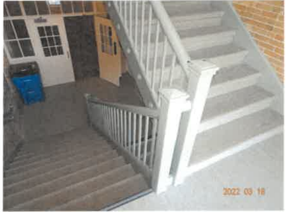
16. View of the stairways.
