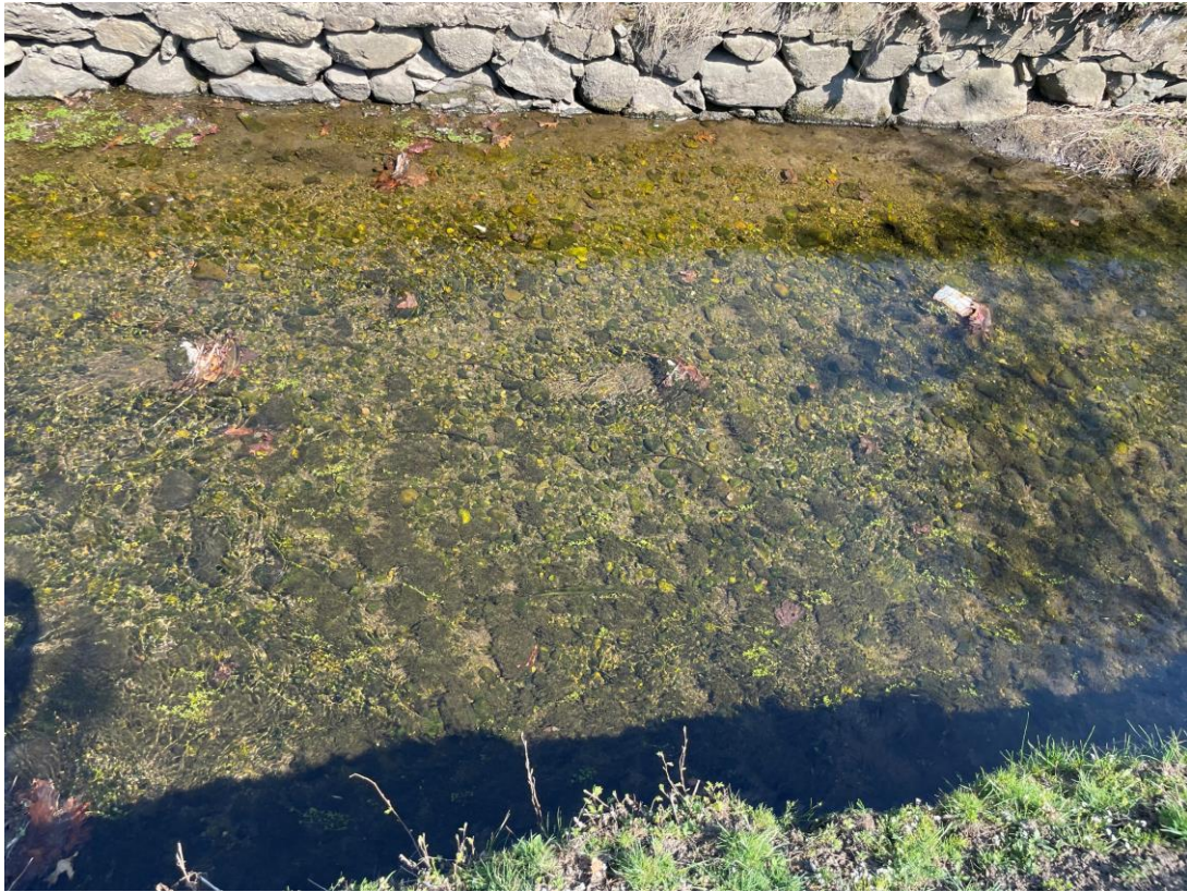
Photo No. 7: View of channel substrate and retaining wall that serves as bank from western bank of Brook. Brook substrate includes gravels and stones and has some algal growth on it.
