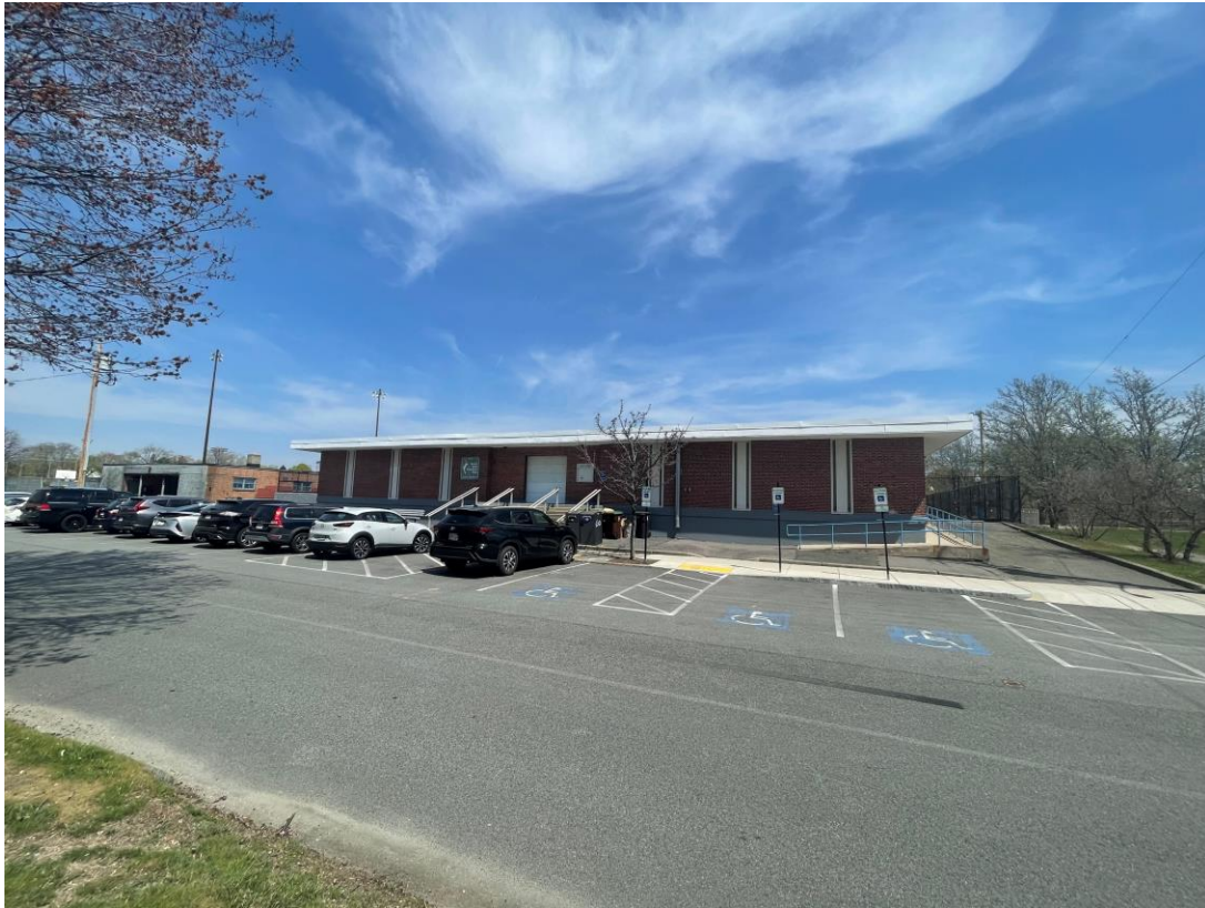
Photo No. 1: View from between Cheese Cake Brook and the building looking east at the building.
