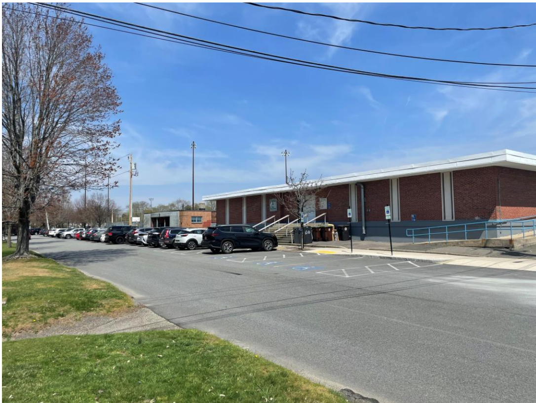
Photo No. 2: View looking north of both buildings on the parcel from southwest of Gath Memorial Pools complex off of eastern bank of Cheese Cake Brook.
