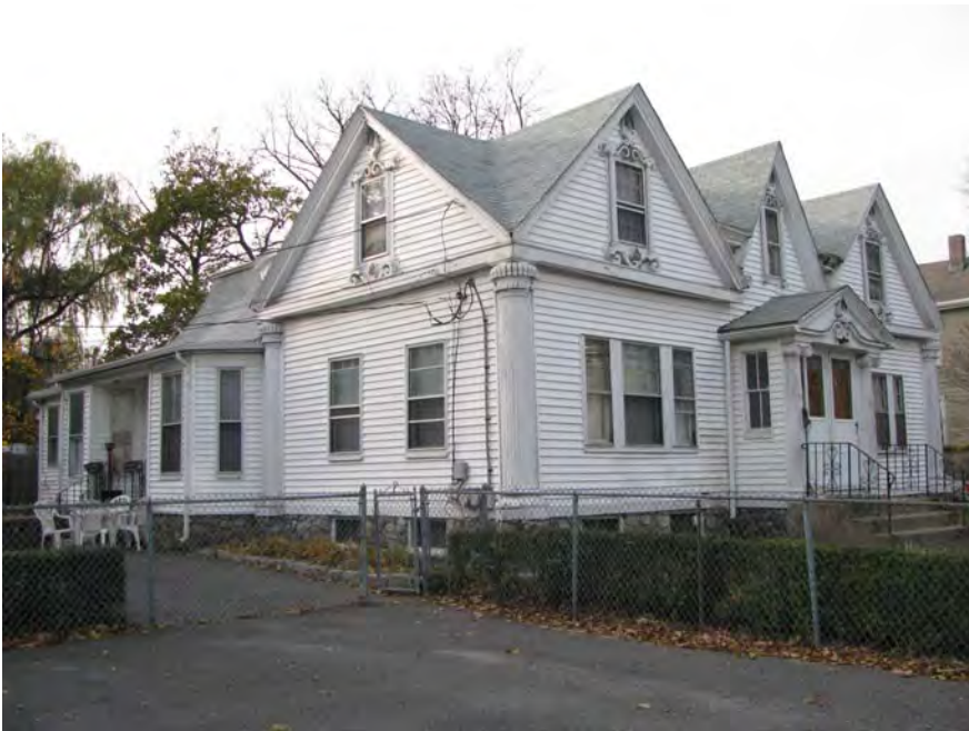
Front / South façade
