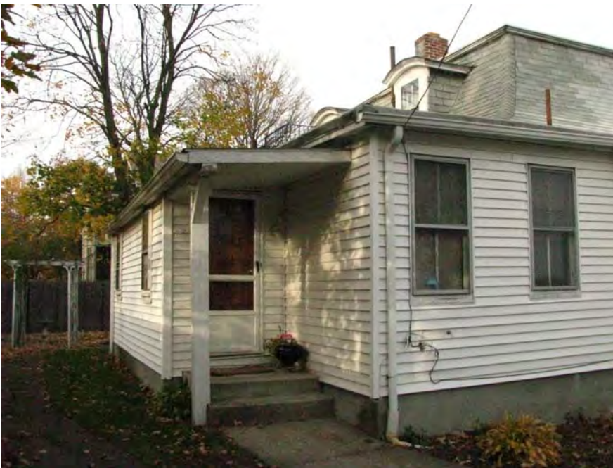
South / Rear façade
