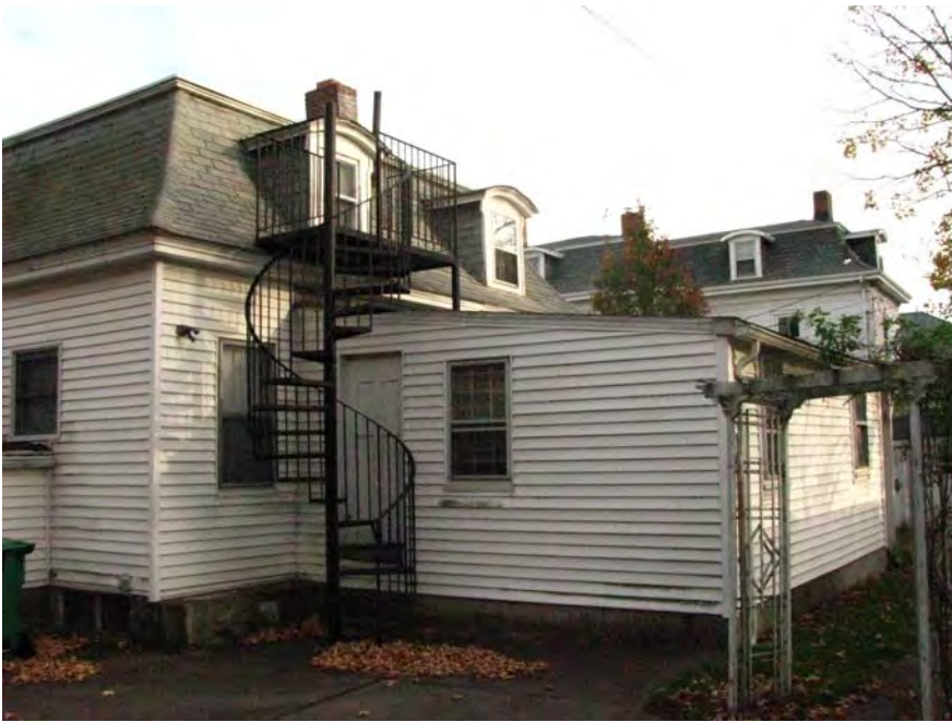
Rear / North facade
