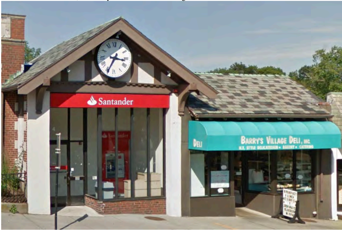
Left to right: Nos. 4 and 6 Windsor Road, from July 2017 Street View image.
