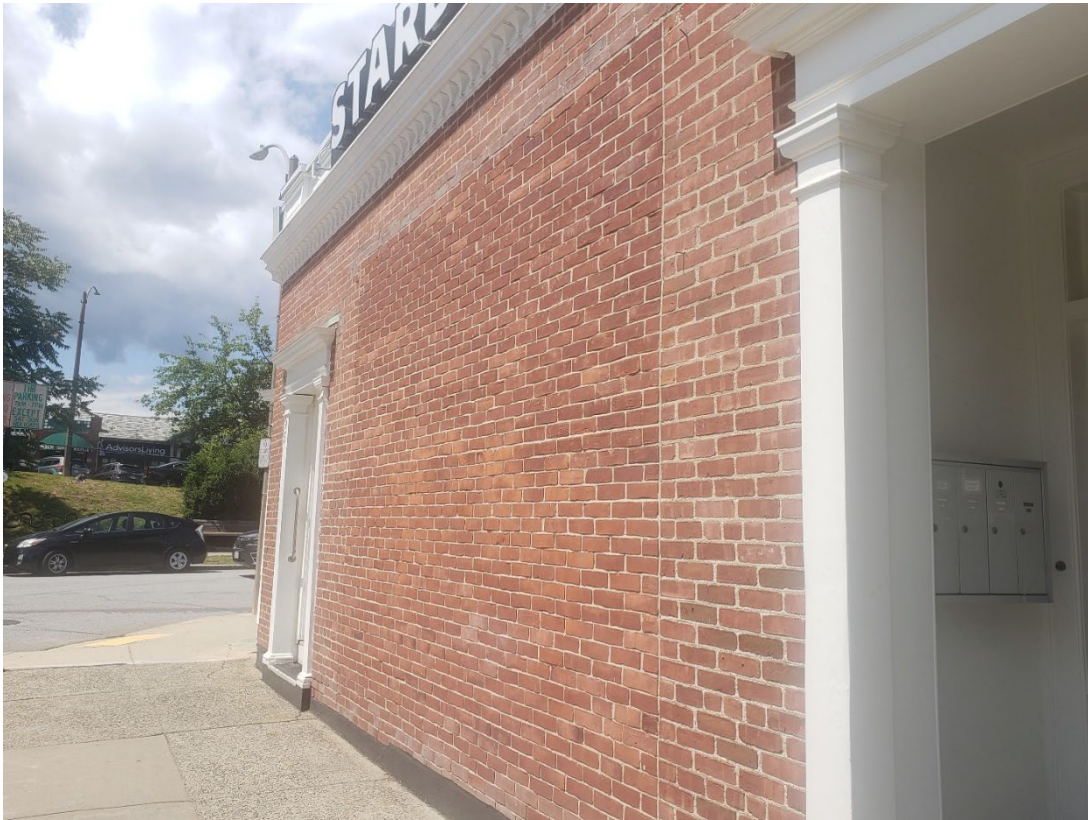
Infill of window on 1933 addition, right elevation
