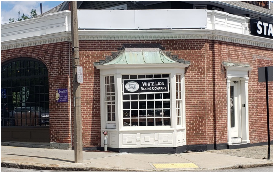
Bay window with copper roof, on corner of front and right elevations
