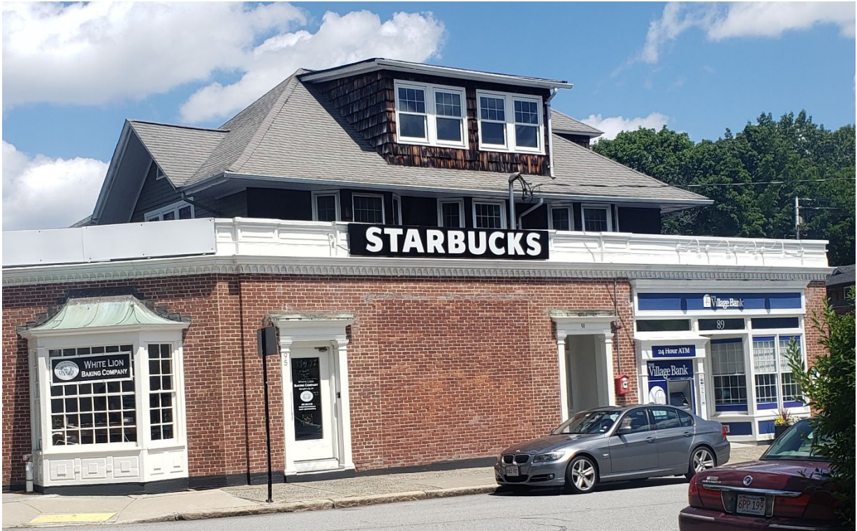
Right elevation, from Waban MBTA parking lot
