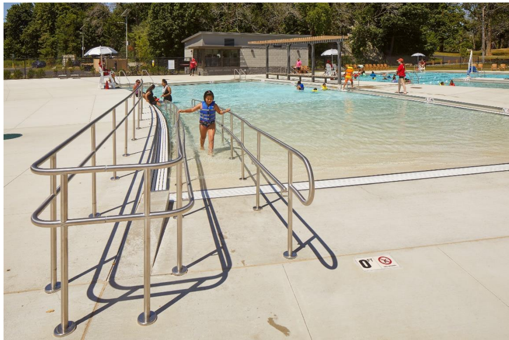
Ramp Access at Zero Depth Entry
