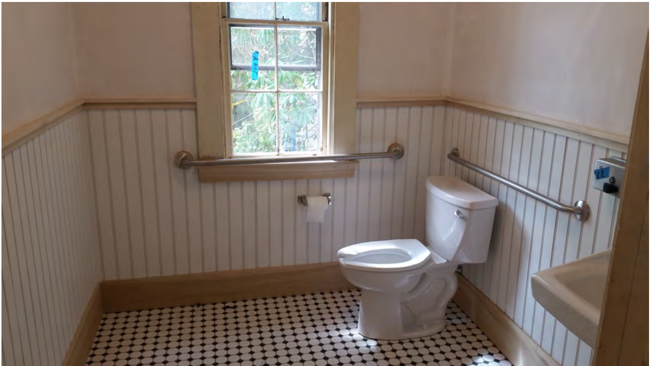
CPC Phase I work: Unisex HC Toilet Room (141)
