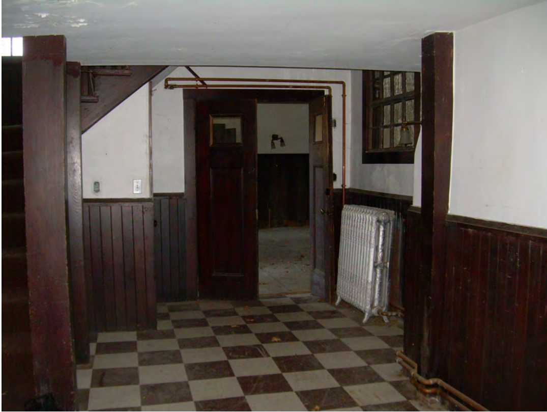
CPC Phase II work: Main Entrance/Lobby (116)
