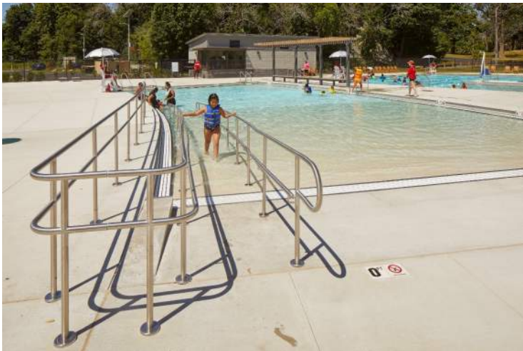
Ramp Access at Zero Depth Entry
