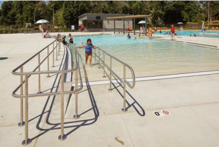
Ramp Access at Zero Depth Entry
