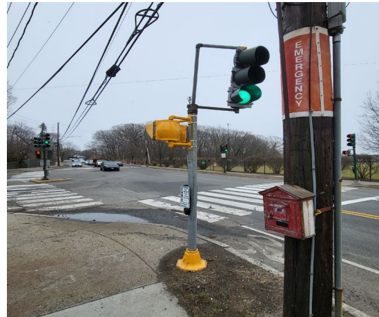
Pictured: Water ponding on the northwest corner of Crafts Street at North Street.
