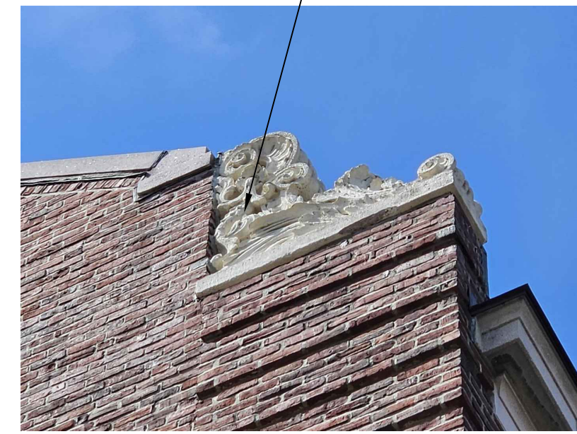
PHOTO 9 - VIEW OF CUSTOM CAST STONE ELEMENTS
