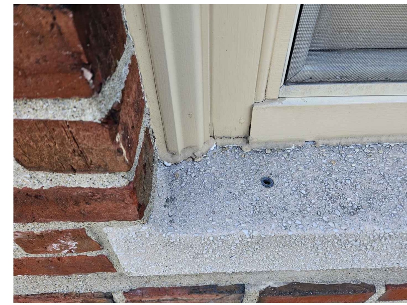
PHOTO 8 - VIEW OF EXISTING WINDOW SILL AND JAMB
