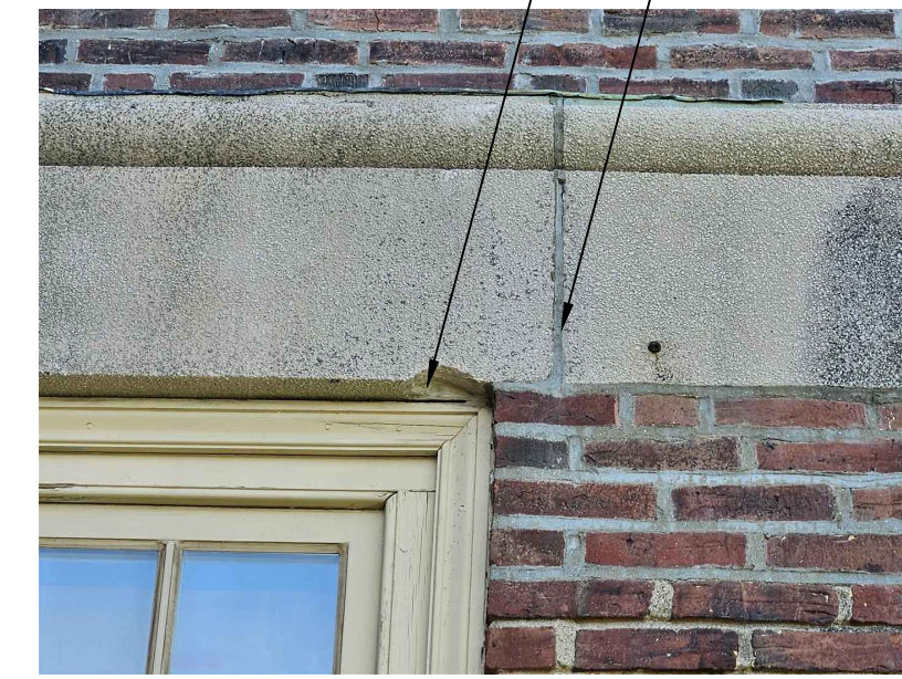
PHOTO 10 - VIEW OF CAST STONE AT LEVEL 1 WINDOW HEAD
