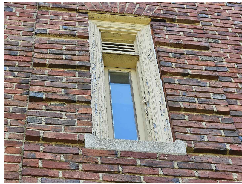
PHOTO 7 - VIEW OF EXISTING DEEP INSET WINDOW WITH LOUVER
