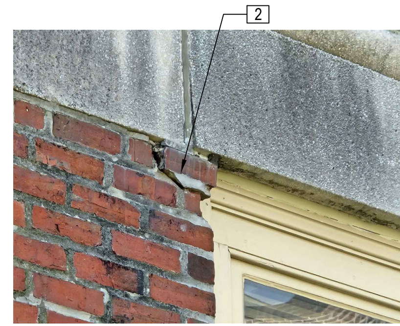
PHOTO 2 - VIEW OF BRICK BELOW CAST STONE
