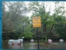
Flooding at Library Parking Lot
