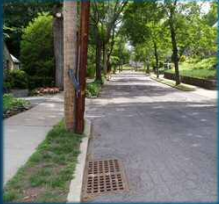
Drainage on Oldham Rd
