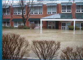
Flooding Near Hammond Brook
