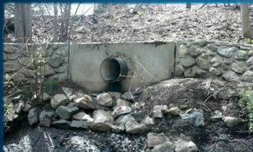
Outfall at South Meadow Brook
