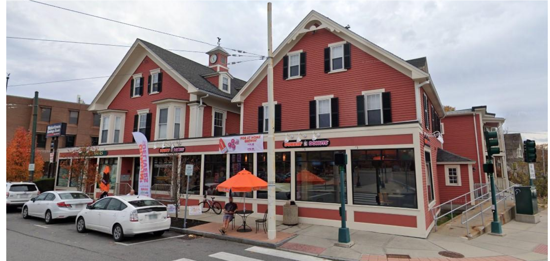
44-54 Church St, Belmont, MA - Ground floor retail with office above
