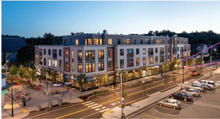
28 Austin Street provides parking that is located behind the building, out of sight from the street
