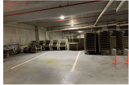
Unused parking from Newton multi-family housing
