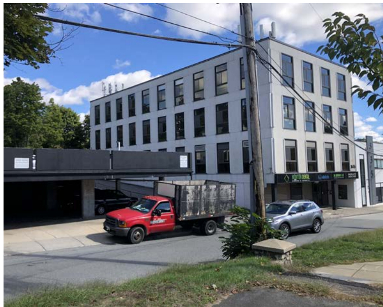
2. View down Jackson St at Route 9
