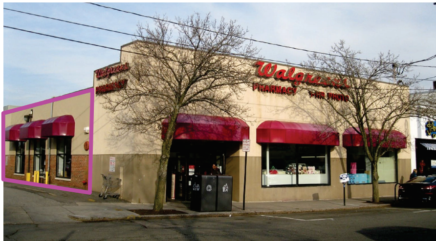
Use located at least 16 feet from the street-facing facade
