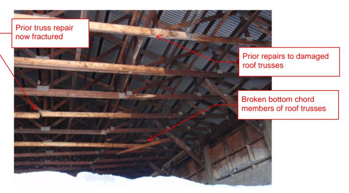
Additional view of bottom of roof trusses. Both buildings exhibited evidence of prior damage to trusses that were repaired with some repairs now failing. Likely causes of damage are strong winds, heavy snow, and long term deterioration of fasteners.
