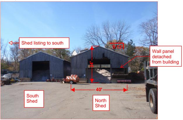
Both structures appear to be experiencing long term deterioration, possibly accelerated from corrosive atmosphere from chloride ions. South shed is listing to the south and several north shed wall panels have fallen away from building (front and sides).
