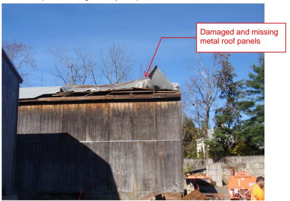
Roof damage at North Shed appears more extensive than South Shed. Sections of metal roof panels are missing or damaged and wood purlins supporting these panels are damaged in several locations. Likely causes are strong winds, heavy snow, and long term deterioration of fasteners.
