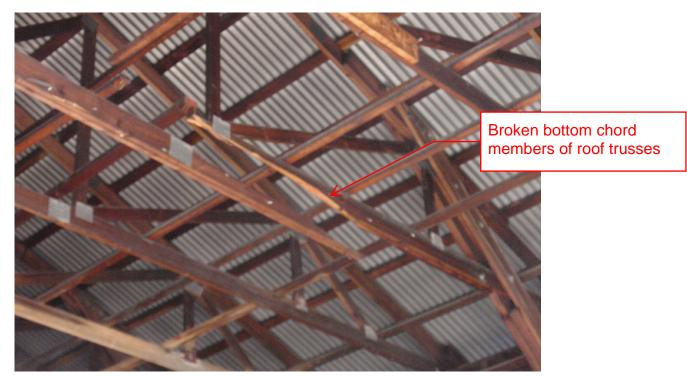
View of bottom of roof trusses in North Shed. Both sheds exhibit similar conditions. Bottom chords are fractured and their capacity is now compromised. Likely causes of damage are strong winds, heavy snow, and long term deterioration of fasteners.
