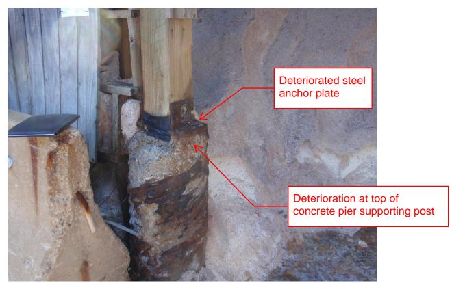
Significant corrosion to concrete piers supporting front entrance. Current condition of piers and anchor plates are significantly compromised from continued deterioration of buildings.
