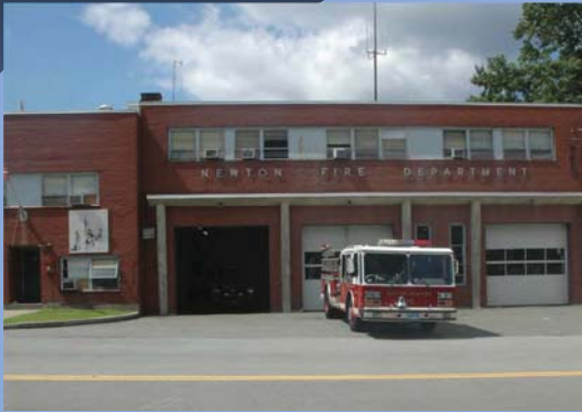
Relocate Wires Division and Replace Fire Headquarters and Station 3
