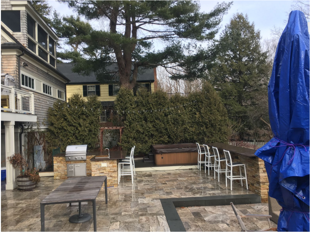
Overview of Existing Paver and Wood Patios, Hot Tub, Arborvitae Hedge, and Pine Tree
