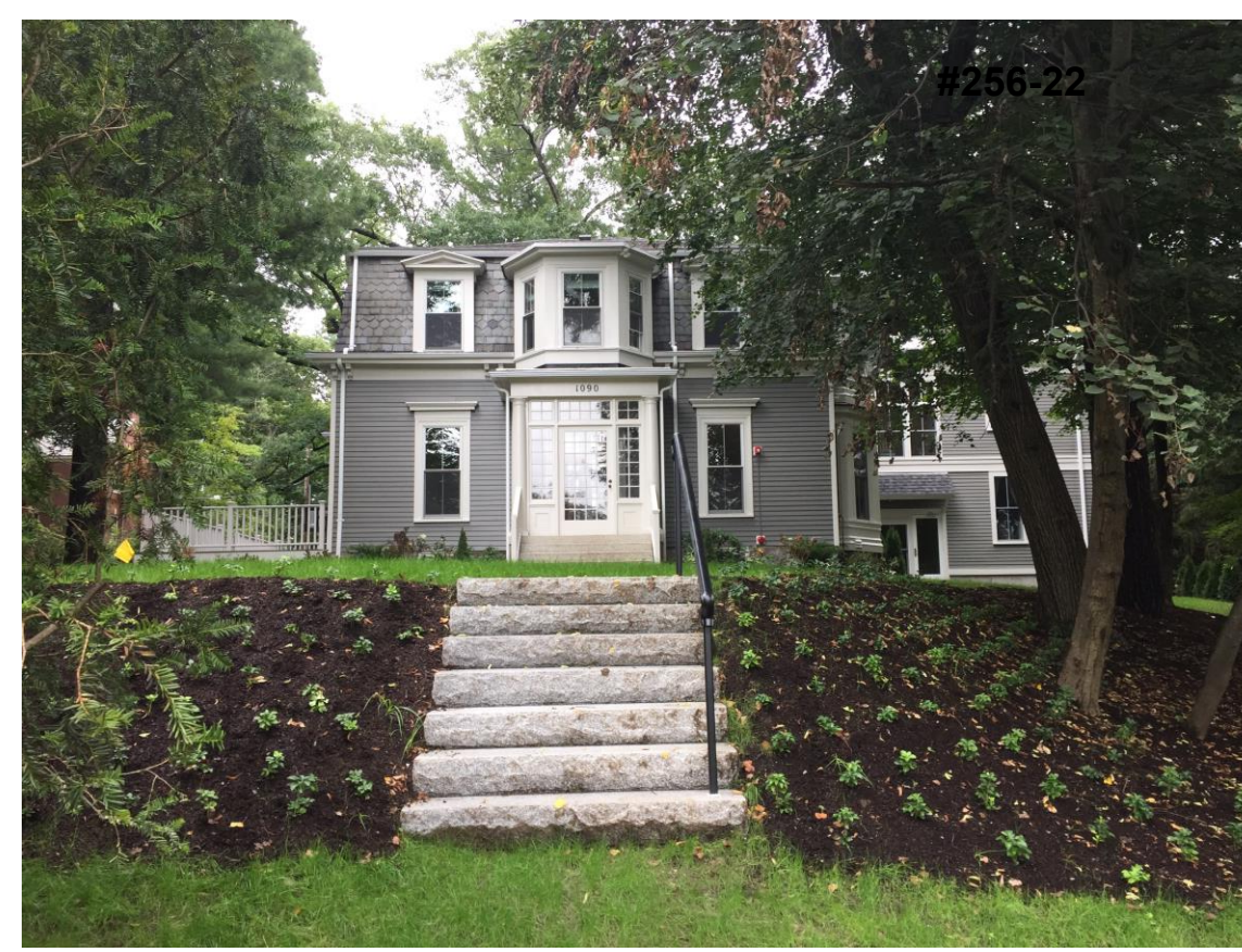
VIEW OF FRONT OF HOUSE FACING WALNUT STREET [SHOWING TOPOGRAPHY]
