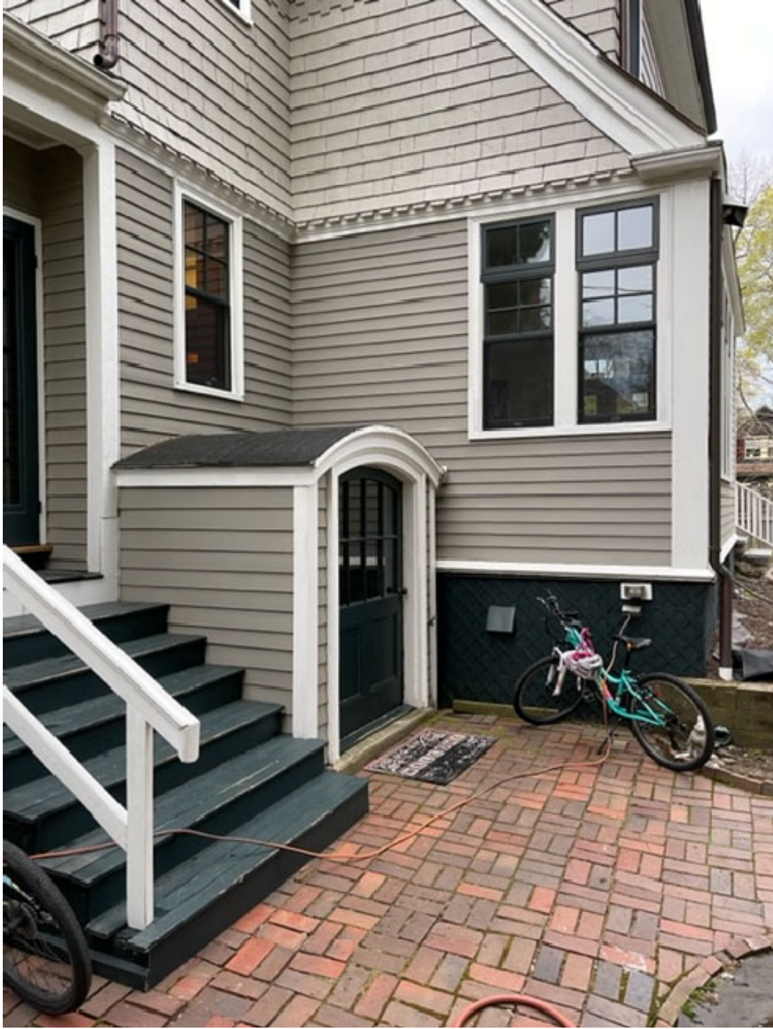
Existing rear corner- future mudroom
