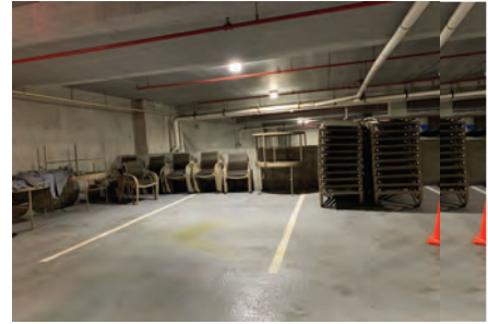
Unused parking from Newton multi-family housing
