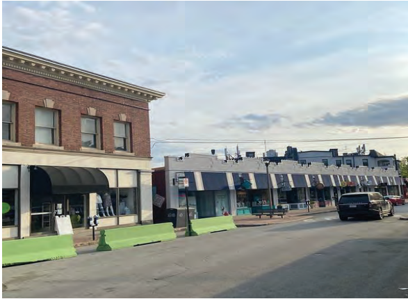
One and two-story retail in Newton Centre
