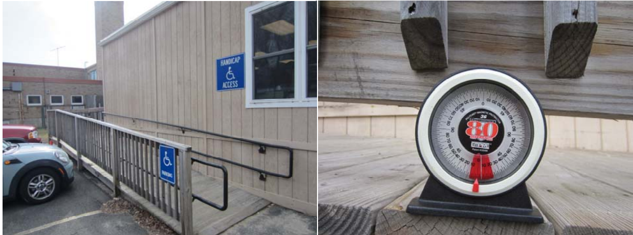
Zervas School – Accessible Entrance
