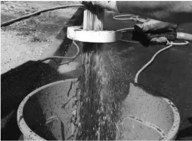
Rinsing Cartridge with Contech Rinse Tool
