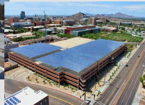
884 kW, Arizona Garage
