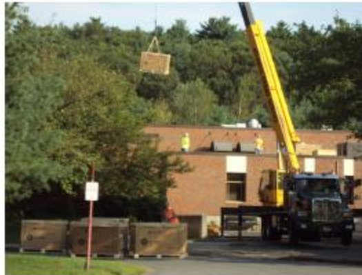
Mobilization & Crane Ops
