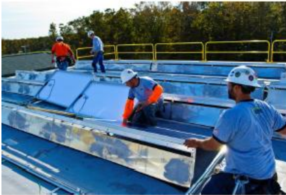
Panel Assembly & Wiring
