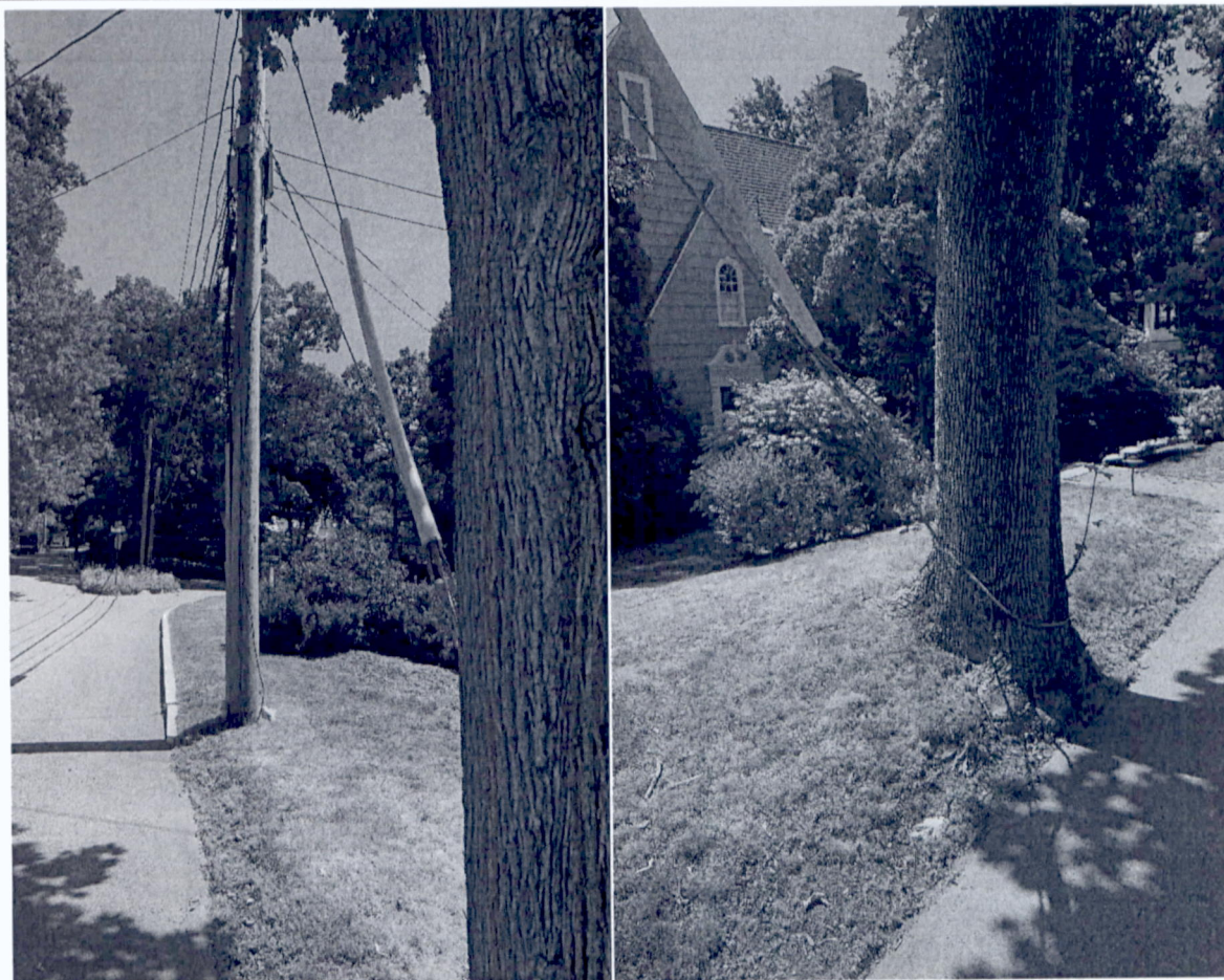
Pole 149/9 with guy wire anchored to a 30" red maple.
