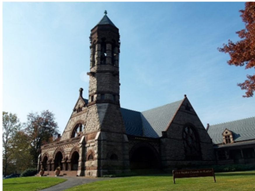
North view of the prominent Bell Tower rising above the building.
