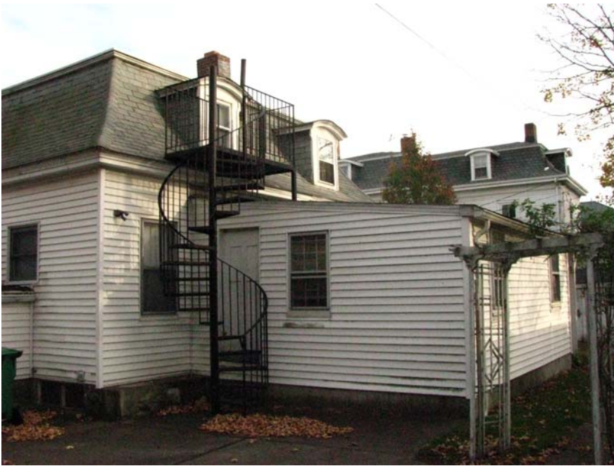
Rear / North facade
