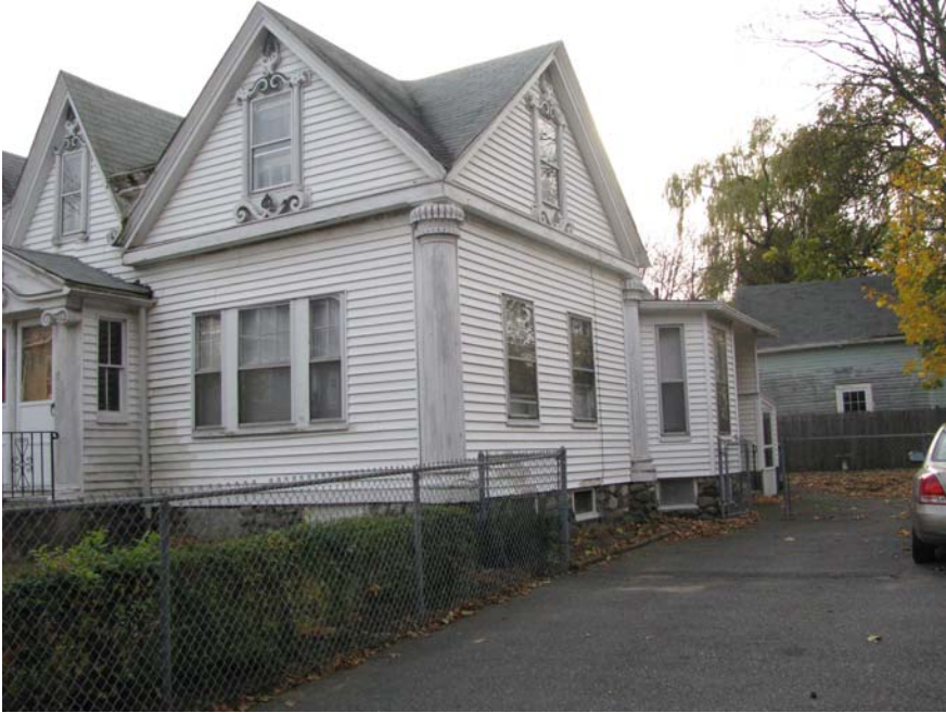
Front / North facade
