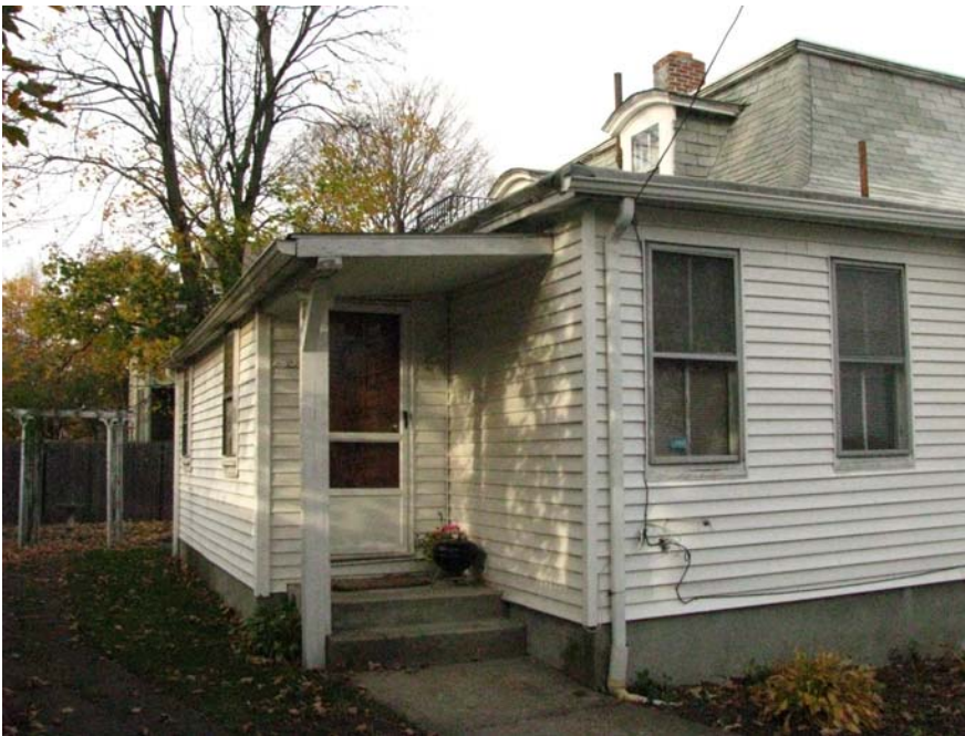
South / Rear façade
