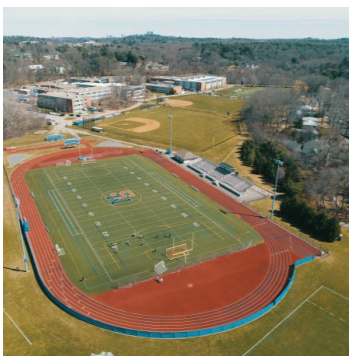
NSHS WINKLER STADIUM LIGHTS (2020)
