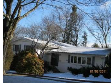
52 Sharpe Road (prior to demolition)
