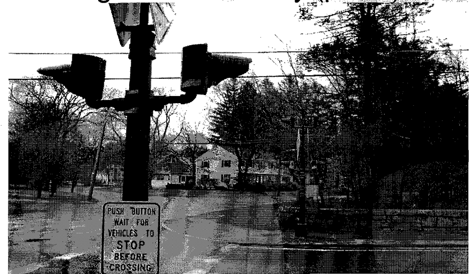
Rt.135 at Amherst Ped. crossing signal in Wellesley (posts)
