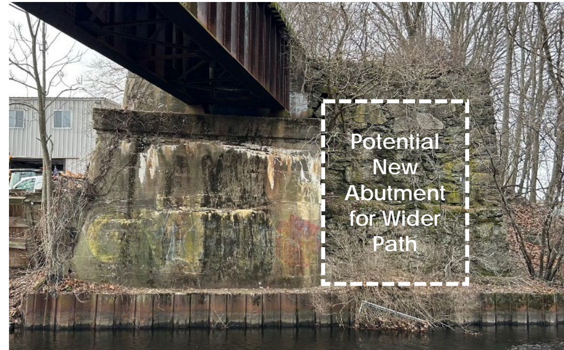
Existing West Substructure
