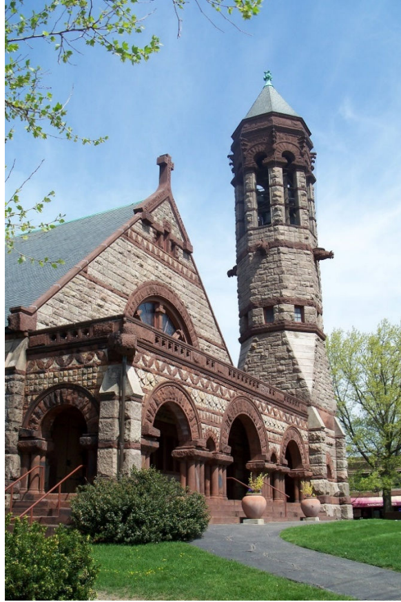
South view of the main entrance and Bell Tower with a clear view of the contrasting colors and shapes of the granite and sandstone stonework.
