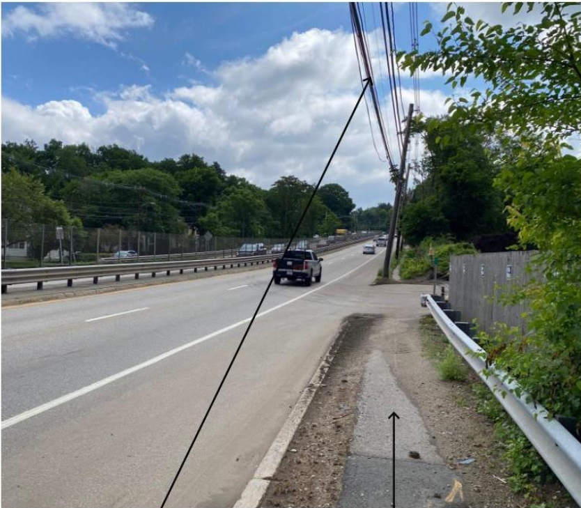
Overhead Utilities Narrow sidewalk with no buffer for pedestrians
