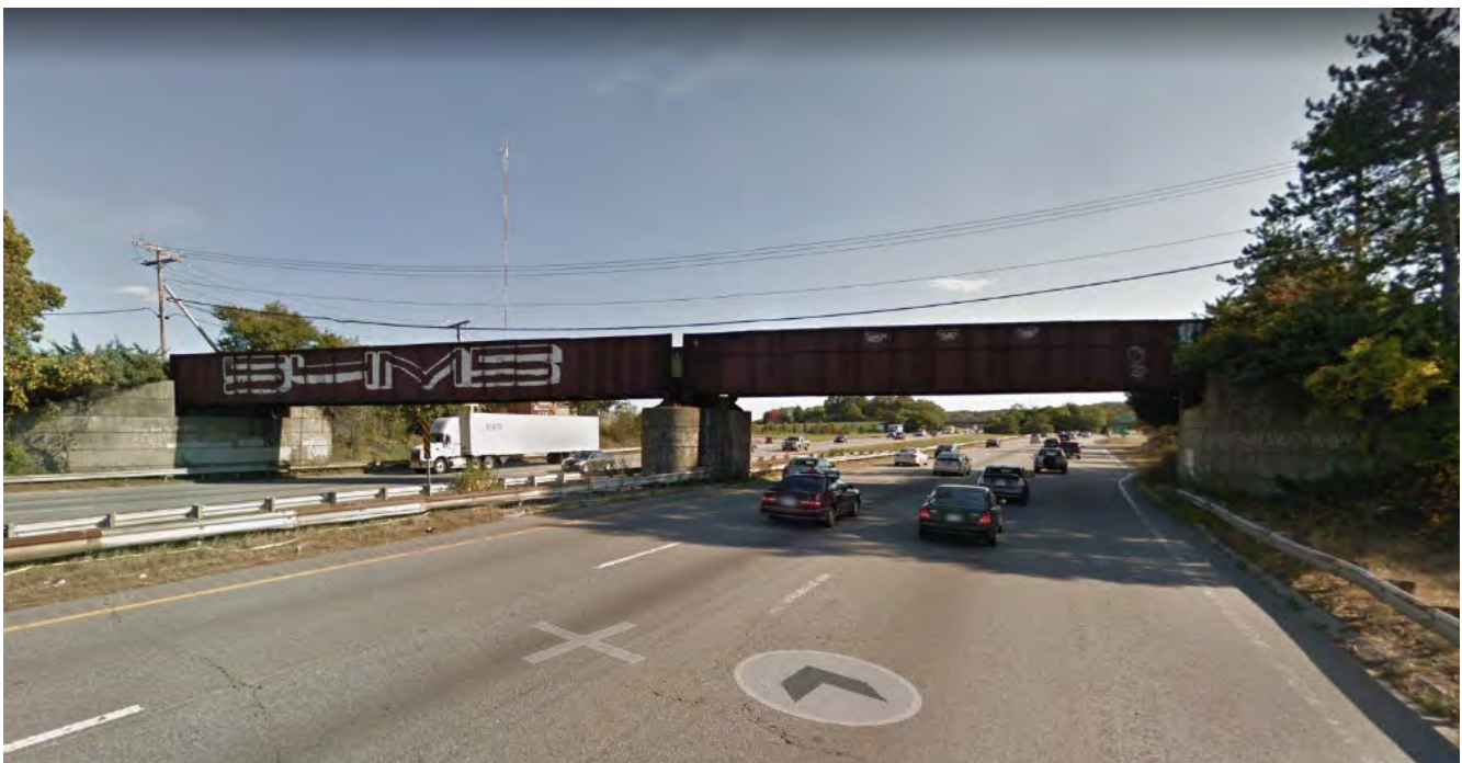
Photo 8: The rail bridge across I-95/Route 128 prior to demolition (Google Earth, October 2011)
