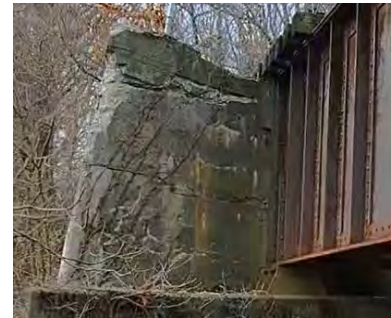
Photo 15: Existing South Bridge Seat
