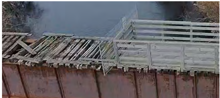
Photo 14: Existing Topside of Bridge
