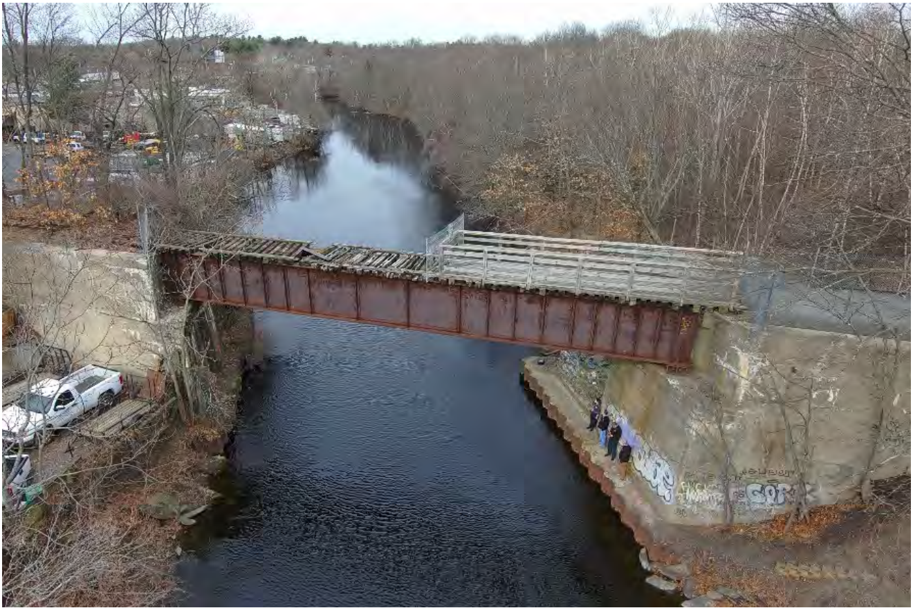
Photo 9: East Elevation of Charles River Bridge (looking northwesterly)
