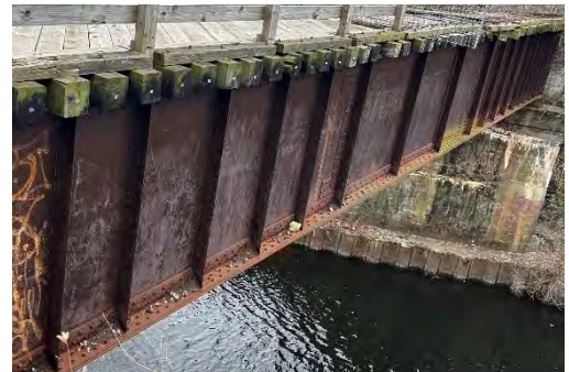
Photo 11: Elevation of West Beam
