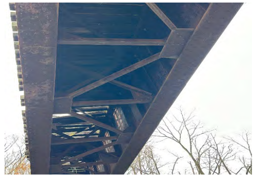
Photo 12: Underside of Bridge
