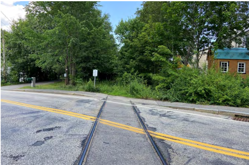
Photo 1: MBTA ROW crossing of Webster Street
