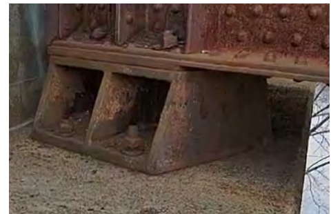
Photo 13: Condition of Bearings
