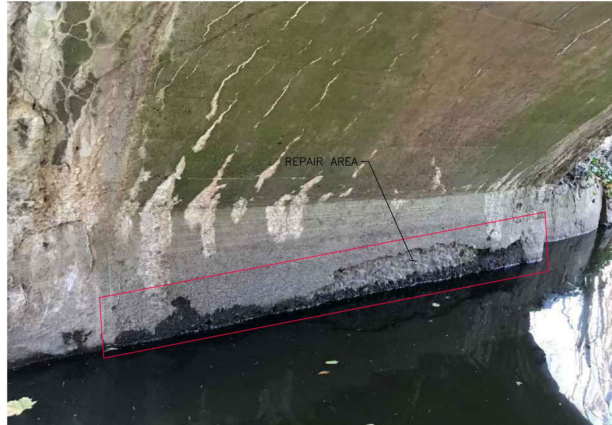
DOWNSTREAM BRIDGE – WEST ABUTMENT N.T.S.
