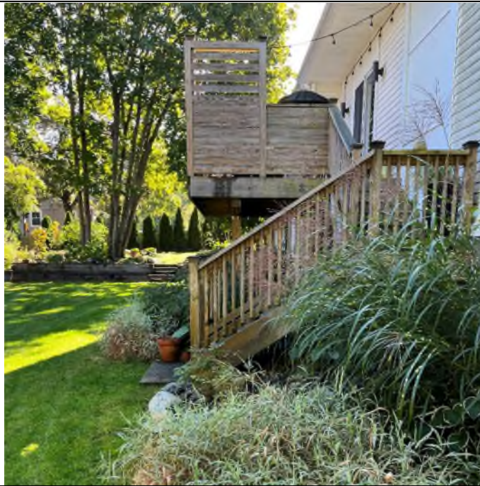
Photo 1. View of existing deck and back of the dwelling, looking east.
