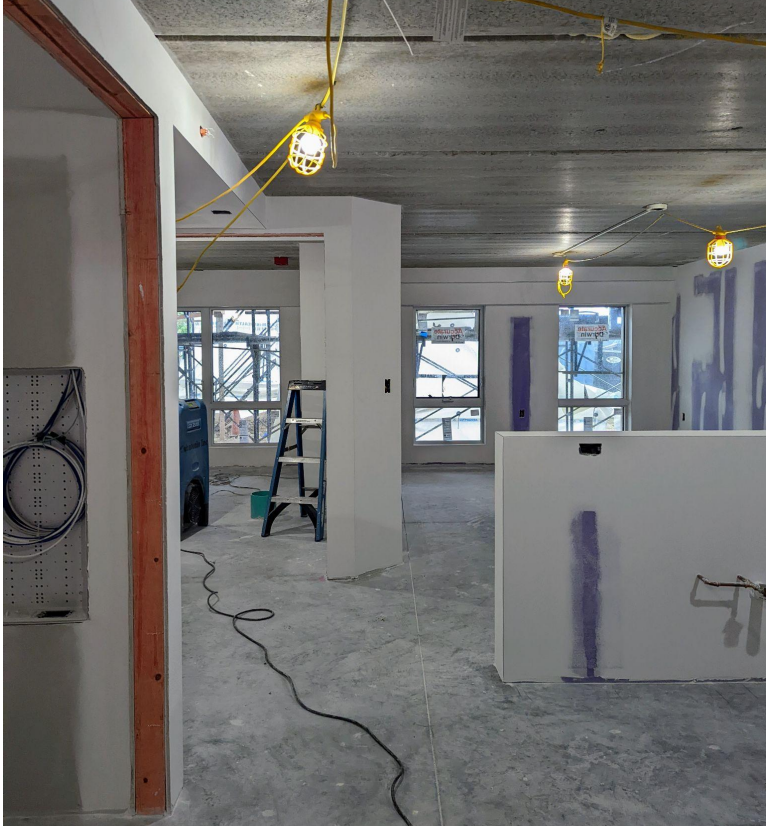
August 23, 2022 Lower addition unit interior drywall
