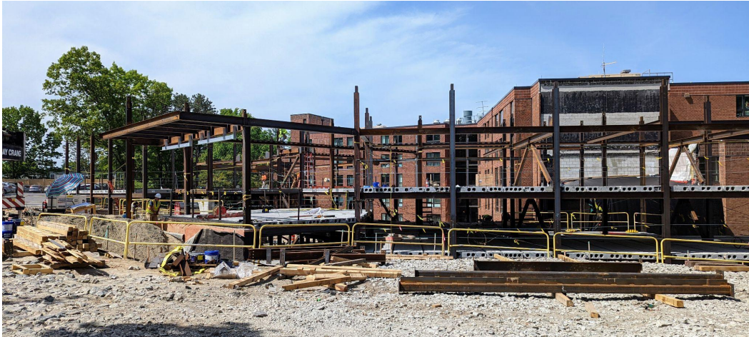
May 24, 2022 upper addition steel framing
