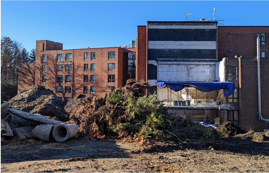
December 7, 2021 Demolition to connect to the upper addition
