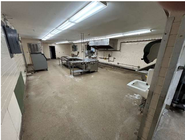
Instructional Kitchen, West Ground floor (5)
