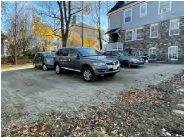
Unpermitted parking lot, view from 128 Washington St
