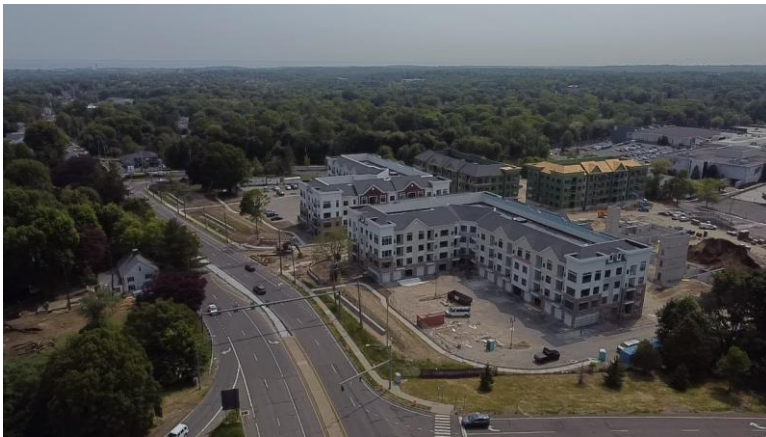
The Residences at Main, Trumbull CT: 260 apartments, under construction
