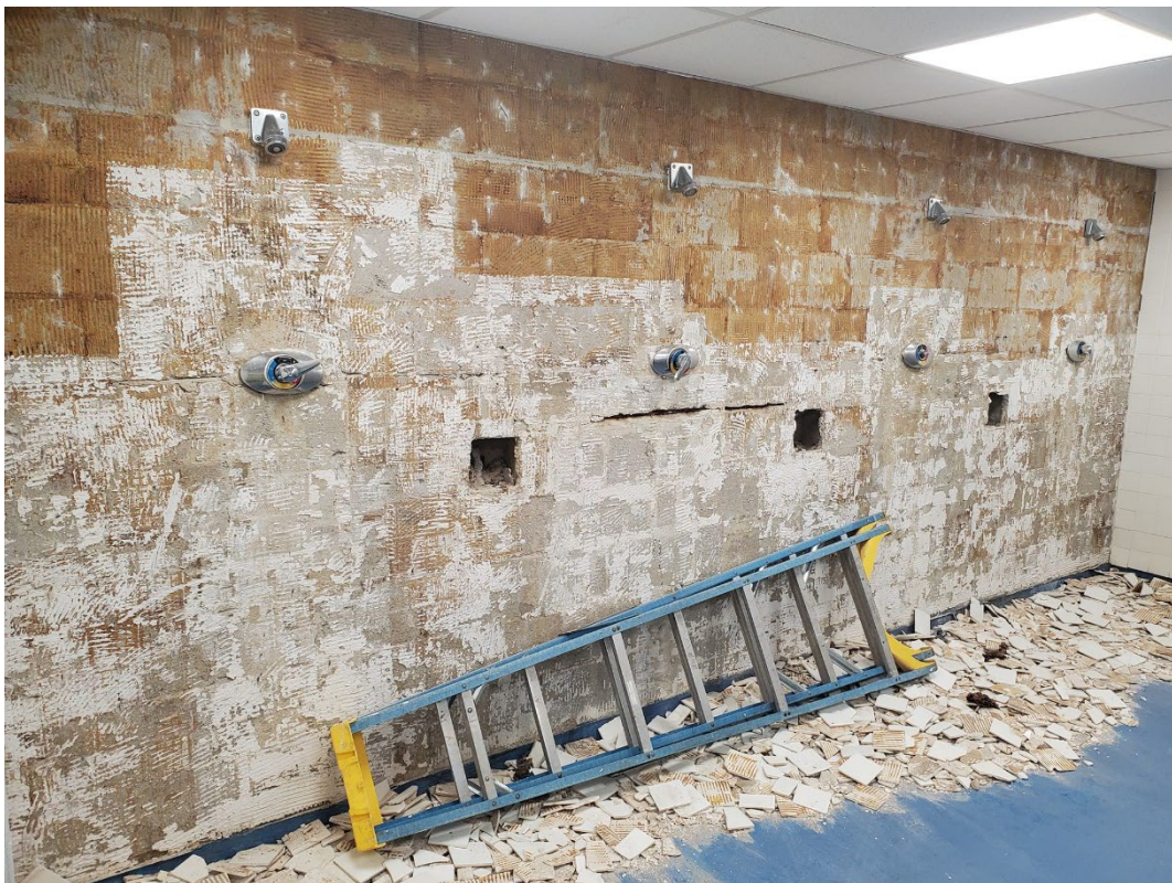
Selective demolition in the restrooms, showers, and locker rooms has started.
