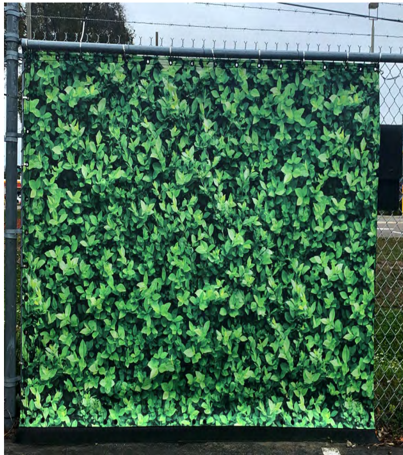
Acoustifence screening along I-90 fence
