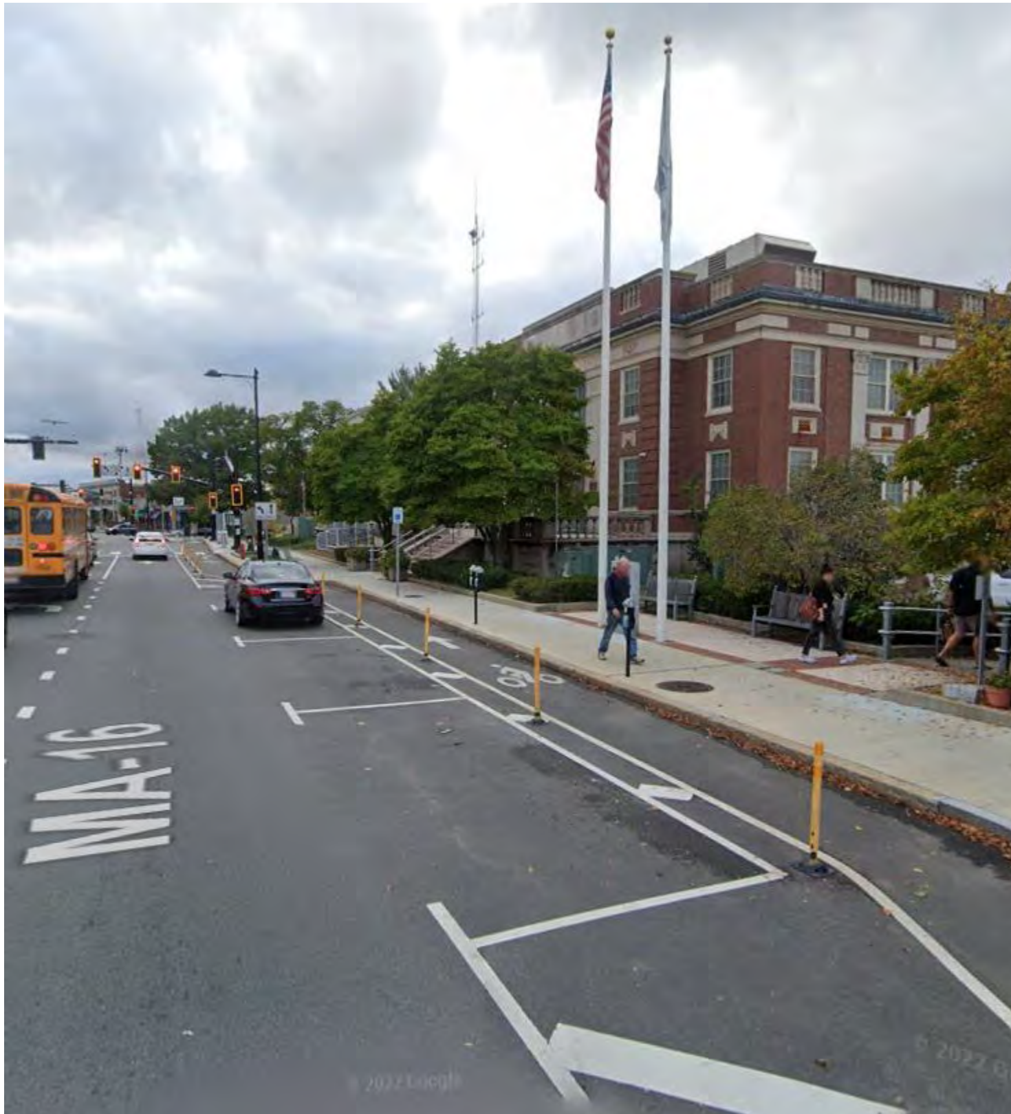
One-way Separated Bike Lanes on North Side of West Newton Square
