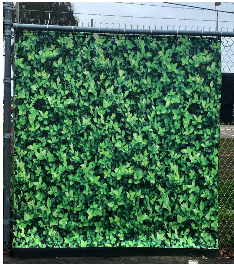
Acoustifence screening along I-90 fence
