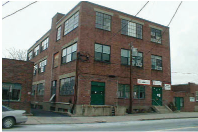
Industrial building on California Street (Manufacturing zoning district)
