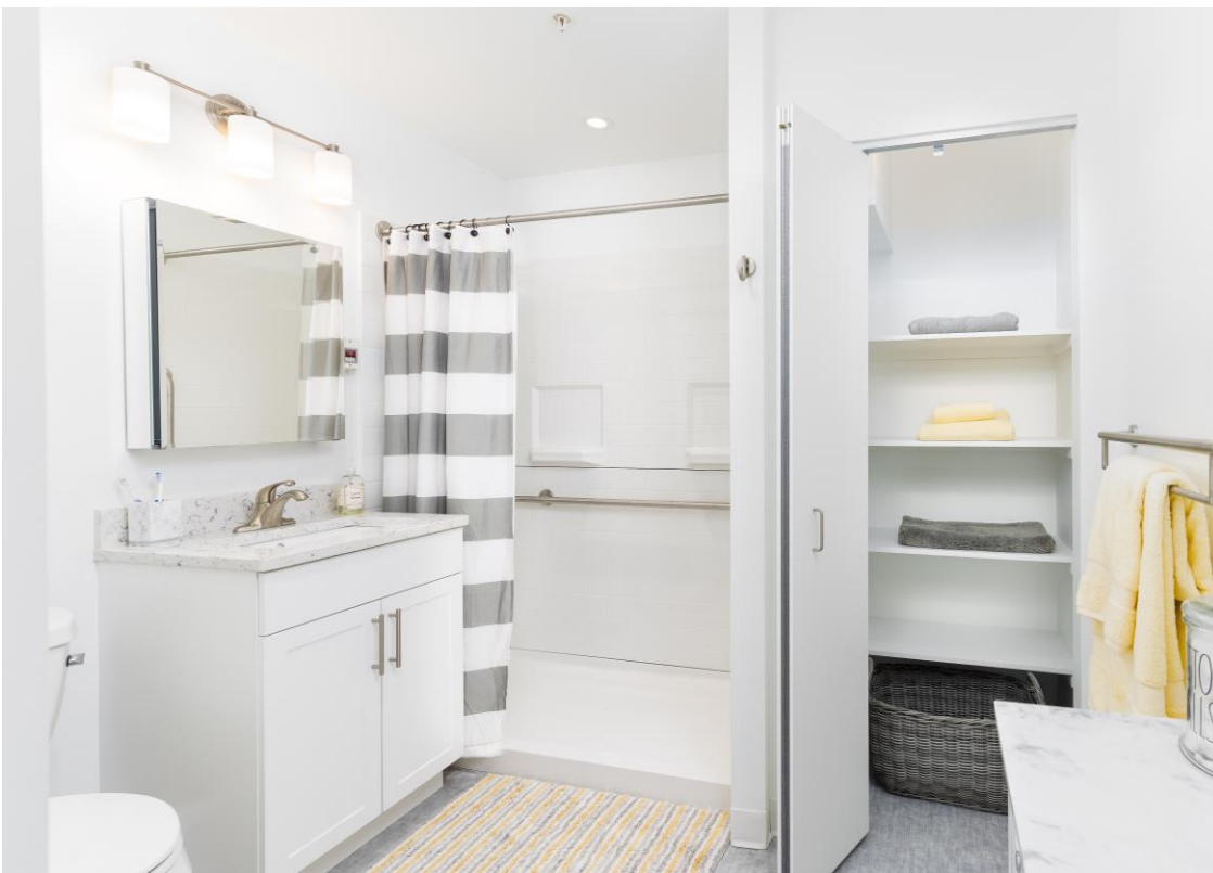
Code compliant bathrooms with turning radiuses and low threshold showers and/or roll in showers depending on existing slab conditions
