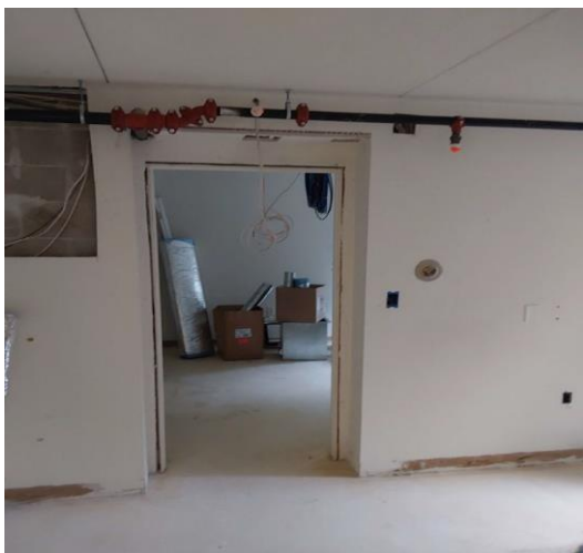
Fully sprinklered apartments
