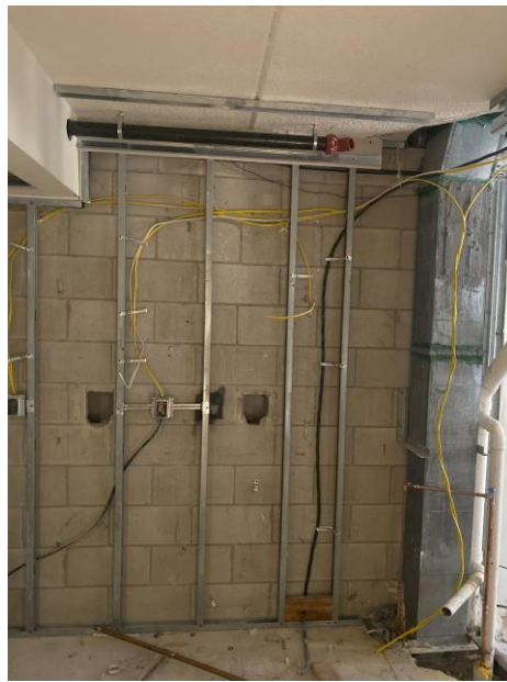
New In-Unit Plumbing and Electrical
