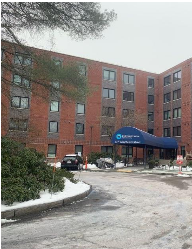
Repaired Façade and New Windows
