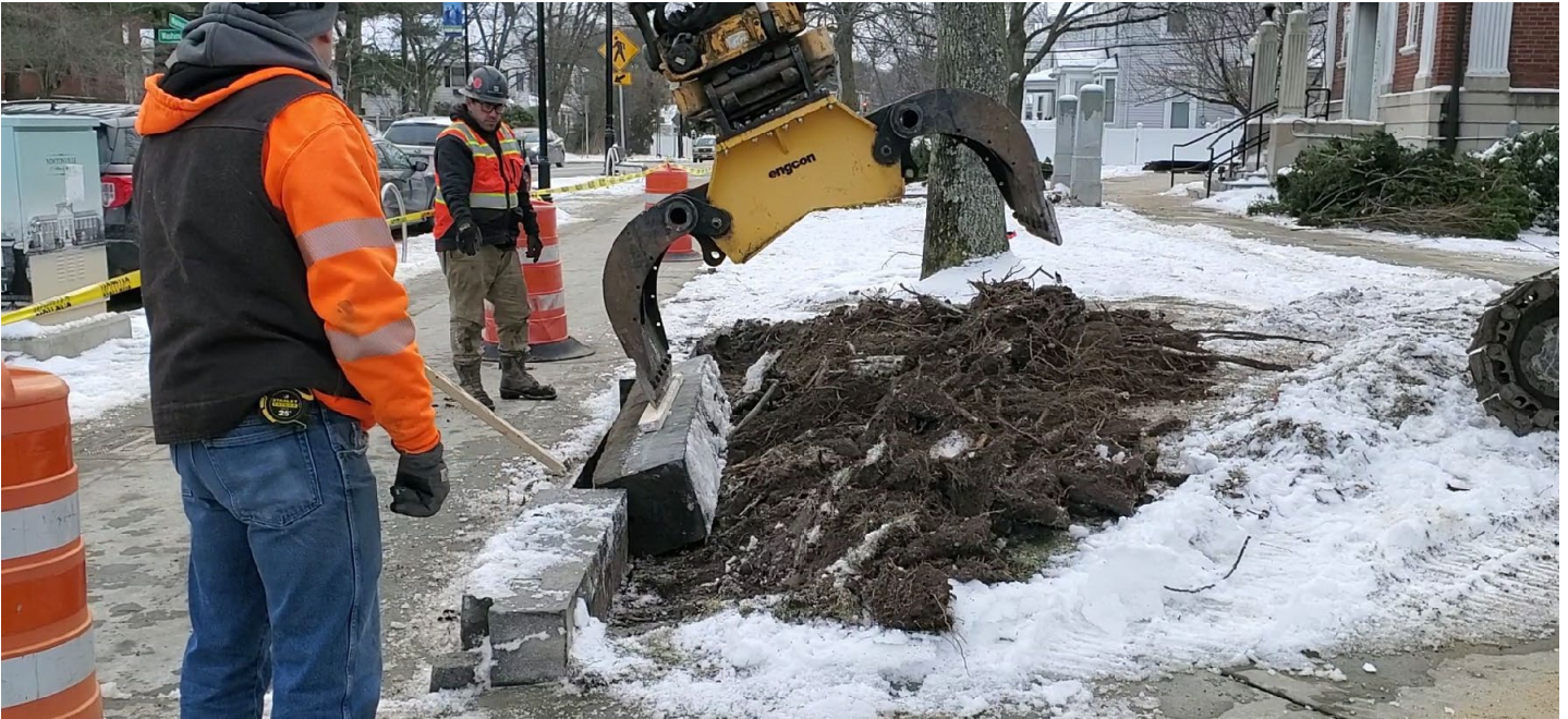
Above - The crews are delicately removing granite elements from around the site. Below the chandelier is being carefully removed for restoration.
